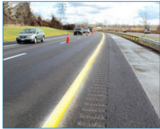
Exhibit 16: Recess Triple Drop pavement markings
