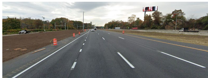
Exhibit 10: The New Rochelle toll barrier was removed as part of a system-wide conversion to All-Electronic Toll Collection, eliminating the need for vehicles to slow, stop, and queue at toll barriers.
