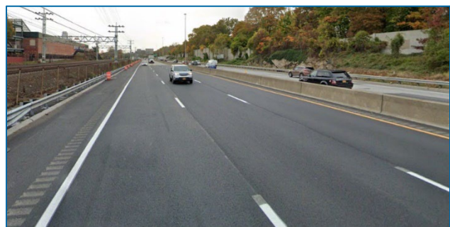
Exhibit 25: Upon completion, the project segment will be in the same condition as another segment of I-95 that was addressed as part of a comprehensive plan to rehabilitate the New England Thruway (I-95) corridor.
