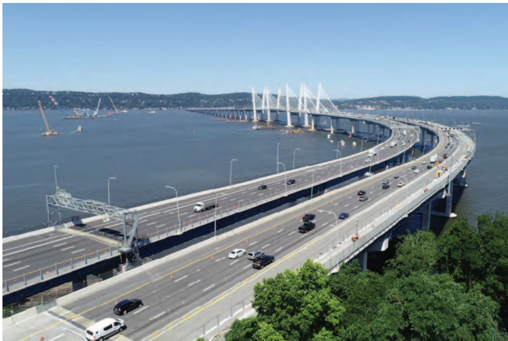
Figure 6: New NY Bridge Project
