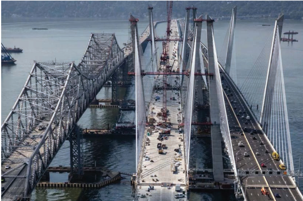
Figure 11: New NY Bridge Project
